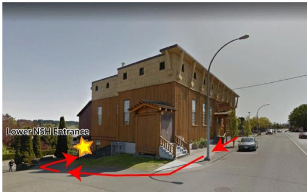
Figure 1: Path of travel for wheelchairs and strollers from the main floor to the lower floor of the Native Sons Hall.
